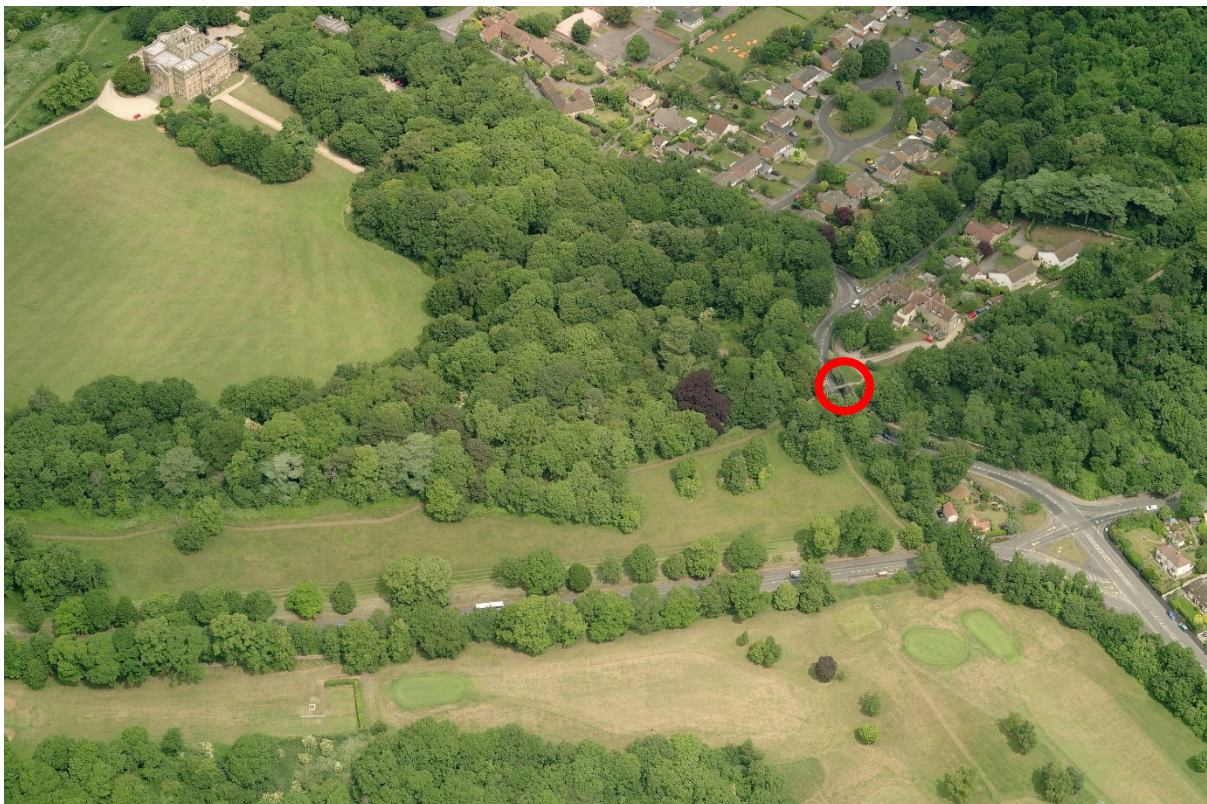
Aerial photograph showing the location of the bridge (highlighted circle) within the wider setting of Kingsweston Estate
